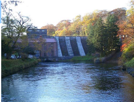
Chitose #4 power plant
