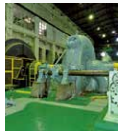
Oji Paper Tomakomai Mill, Chitose No. 1 Hydroelectric Power Plant (Inside)
