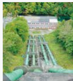
Oji Paper Tomakomai Mill, Chitose No. 1 Hydroelectric Power Plant
