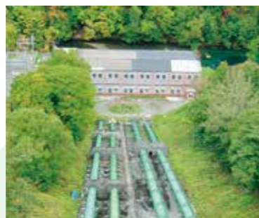
Hydroelectric power plant
