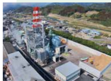
Biomass power generation
