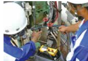
An energy conservation control at the Oji Paper Kasugai Mill. The patrol confirms that there is no waste caused by air leaks.
