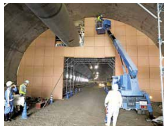
New construction method using HiPLE-ACE
