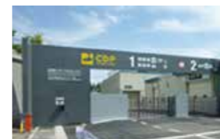
Confidential document processing facility (Oji Materia Co., Ltd. Edogawa Mill)
