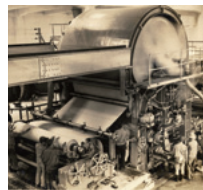
#1 machine at Kasugai Mill
