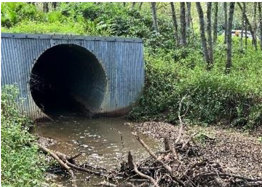
River structure (e.g., culverts) improvements and re-meandering small rivers
