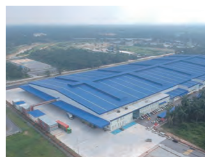
Tenth corrugated container plant in Malaysia
