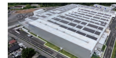
Solar power generation facility at Tochigi Plant, Oji Container
