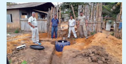
Septic tanks donated to third parties
