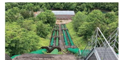
Chitose No. 1 Hydroelectric Power Plant
