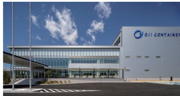
Integrated plant for corrugated containers in Tochigi Prefecture (started operation in February 2023)
