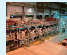
#12 machine prior to its relocation
