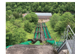
Tomakomai Mill-owned Chitose No. 1 Hydroelectric Power Plant
