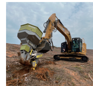
Automatic planting machine during plowing-in operations
