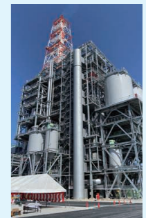
Oji Green Energy Tokushima started operation of biomass power plant in Tokushima Prefecture. (P58)
