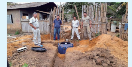
Septic tanks donated to third parties
