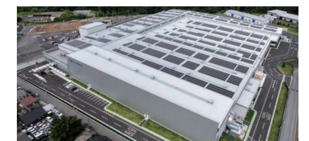
Solar power generation facility at Tochigi Plant, Oji Container
