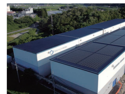
New film machine building at Oji F-Tex Shiga Mill
